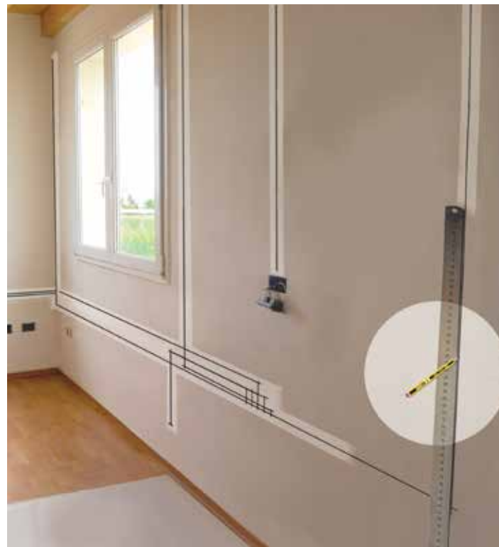
Step 1. Drawing the electrical tracks on the walls to lay Next .
